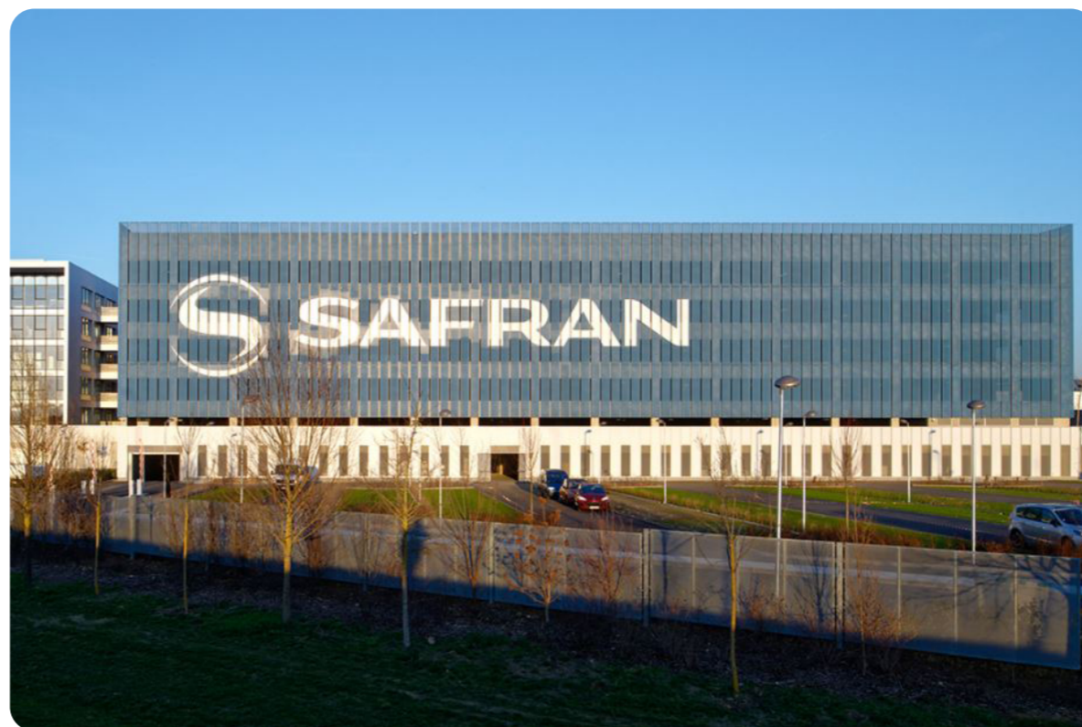
Safran Car Park | Blagnac - Toulouse - France - 4000 m 2
